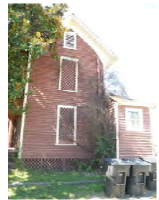
Figure 4 South elevation of end of building
