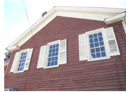
Figure 23 Windows and shutters on the northeast elevation
