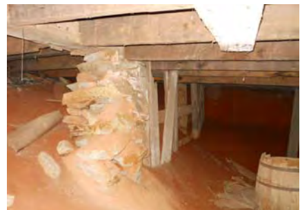
Figure 19 Stack stone foundation
