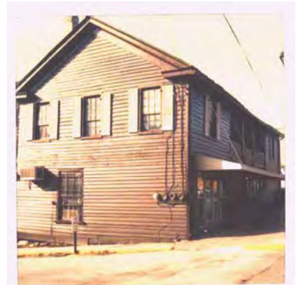
#16. c1860 Rev. Goodman Hughes House E. Main St. Dahlonega, Ga. Mar 1982
