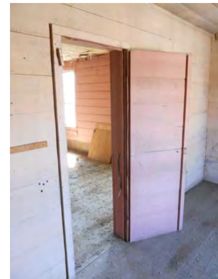
Figure 22 Interior doors vary in size and construction and were built for each opening.
