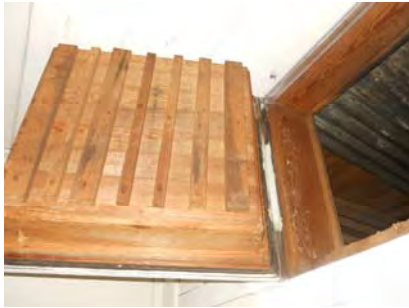
Figure 12 Door to ice chamber above cold storage
