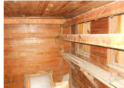
Figure 14 Cold storage space with hooks and shelves for meat storage
